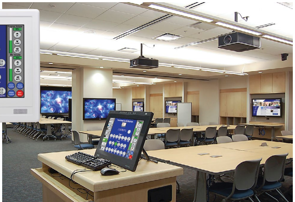
One of the podiums with a keyboard and monitor for an instructor workstation, which allows the instructor to access the room controls (see inset).
