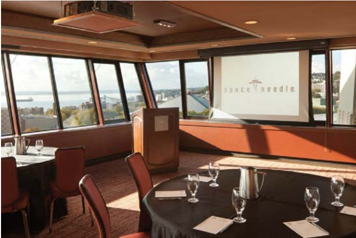
The system uses 6000-lumen Panasonic PT-DZ6700U high-definition projectors with the Chief projector lifts and Da-Lite Tensioned Contour Electrol screens already installed the tower's three meeting rooms. An all-digital AV system on a Crestron DigitalMedia backbone assists in The Skyline Center's hosting 30 to 50 events each month, ranging from corporate directors' meetings to training sessions, weddings, and holiday parties.
