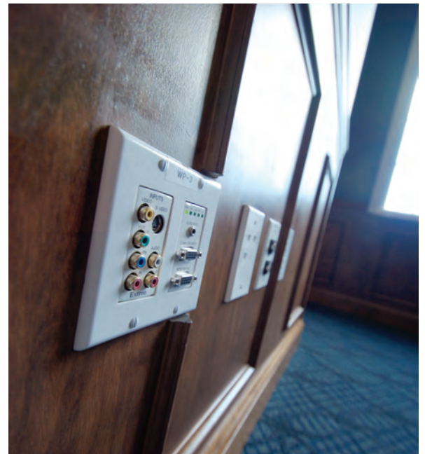
Above: Digital signage monitor outside the ballroom shows the day's schedule. Top right: AMX panel in the control room. Below left: The ballroom, an ABC combinable room, with air walls open. Below right: Extron wall plate with component, S-Video, VGA, and audio inputs plus VGA monitor out.
