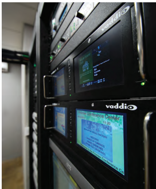
Left: The signage head end in the control room. The signage system is powered by a Keywest MediaZone server, which can send messages to an LCD panel in the lobby, another outdoors, and to each of the meeting rooms. Above: The 64x64 Extron Cat-5 switcher, which routes any signal from any source to any combination of displays and sound systems in the facility.
