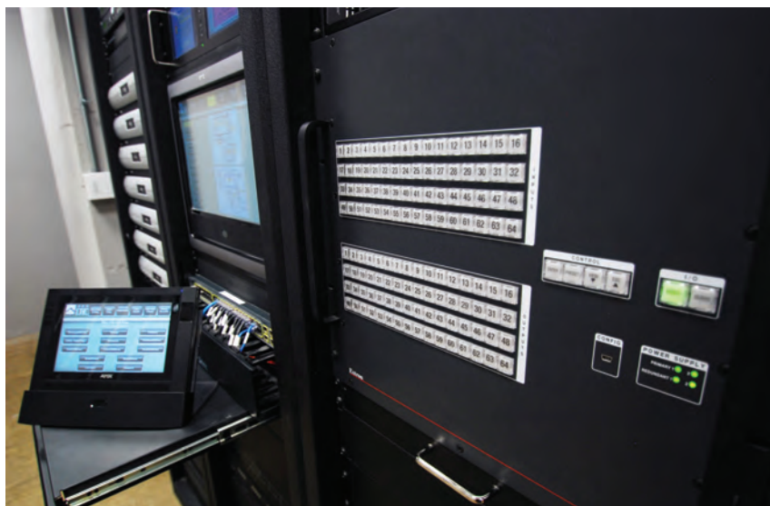
Left: The signage head end in the control room. The signage system is powered by a Keywest MediaZone server, which can send messages to an LCD panel in the lobby, another outdoors, and to each of the meeting rooms. Above: The 64x64 Extron Cat-5 switcher, which routes any signal from any source to any combination of displays and sound systems in the facility.
