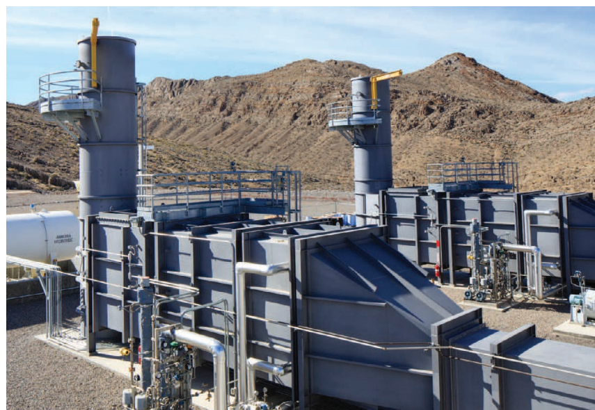
Selective catalytic reduction (SCR) are typically found on large gas turbines to reduce NO x by 70-95%
